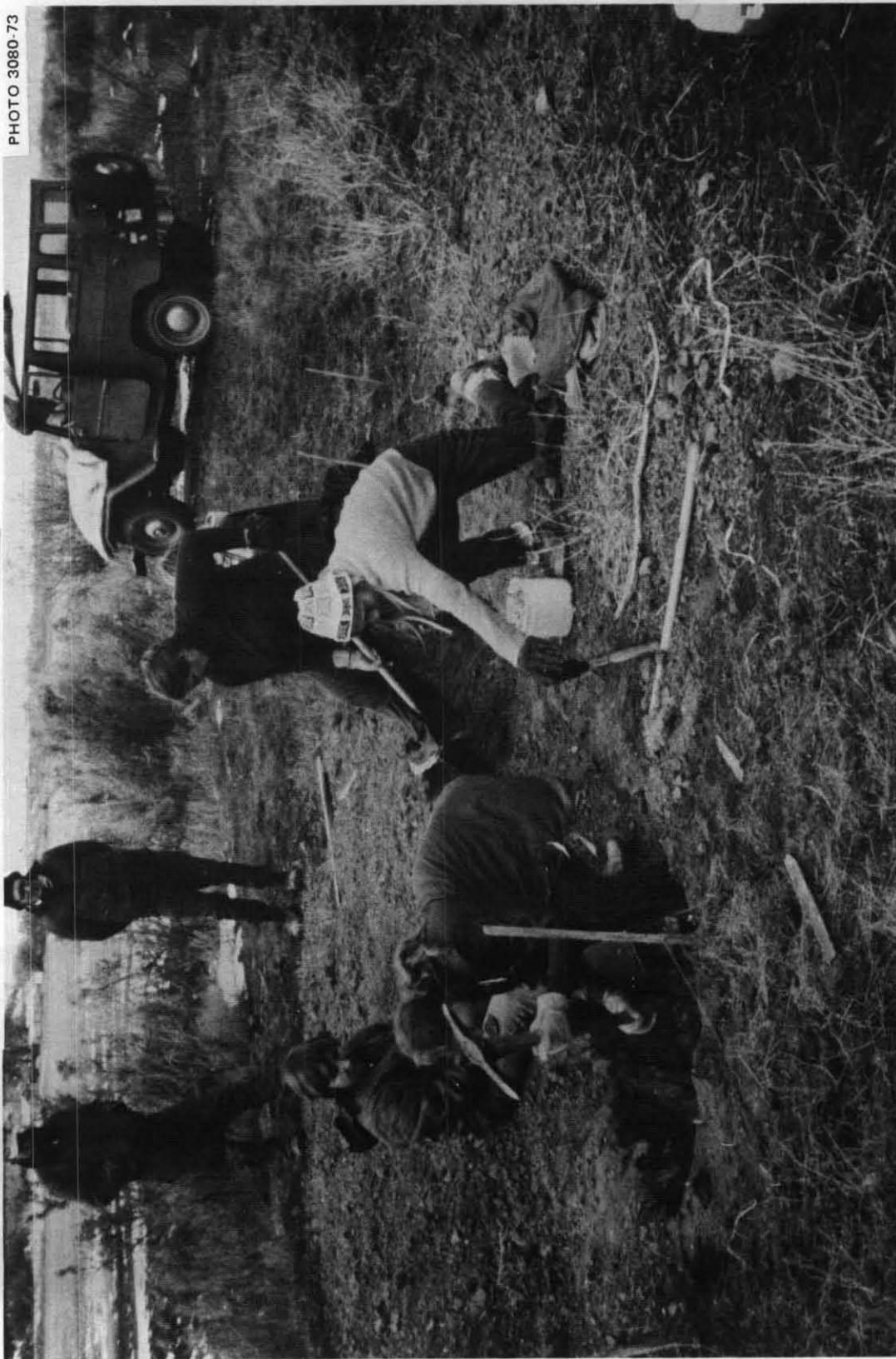
Fig. 2.3. The mother dug inefficiently with her dull shovel with pushing it with her foot. She dug the trench too narrow until it was almost completed – in spite of having read the instructions to the contrary. Until the second day, no member of this family learned to swing their dull old pick properly, by letting one hand slip toward the other as the pick descended. Nor did they know how to use their other tools properly.
